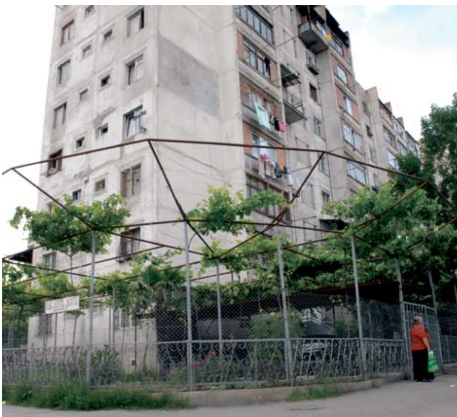
Garden canopy construction. Gldani, Tblisi
